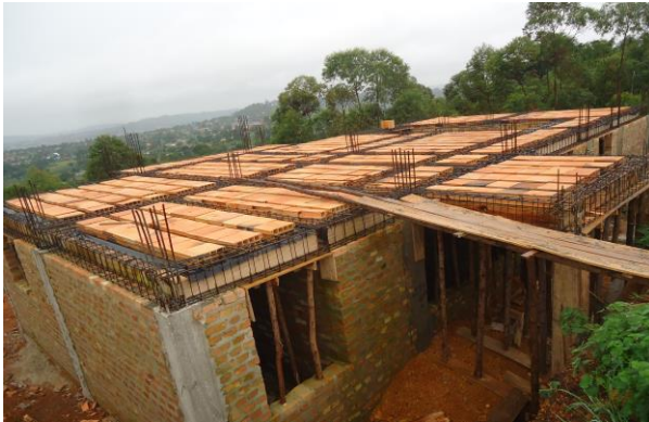
Prime Radio broadcasting house under construction in Masaka
